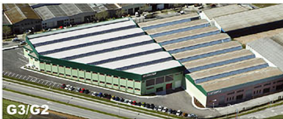
FACTORY GIRBAU 2: heavy-duty laundry equipment (batch washers, presses, dryers, conveyors, etc.)
