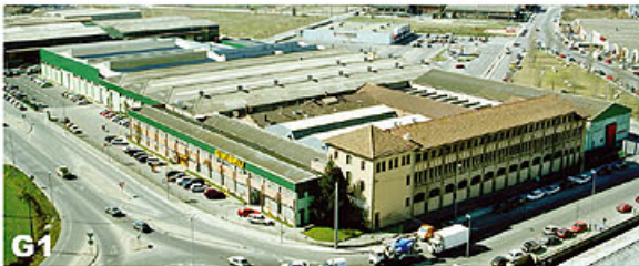
FACTORY GIRBAU 1: washer extractors and flatwork ironers
